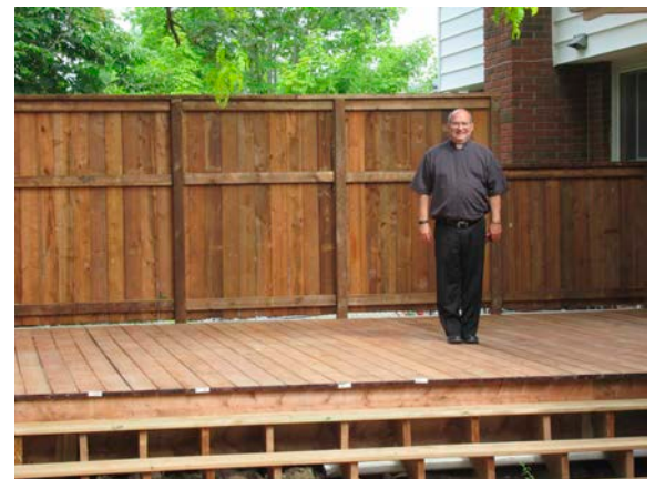
New Deck at the Rectory!
